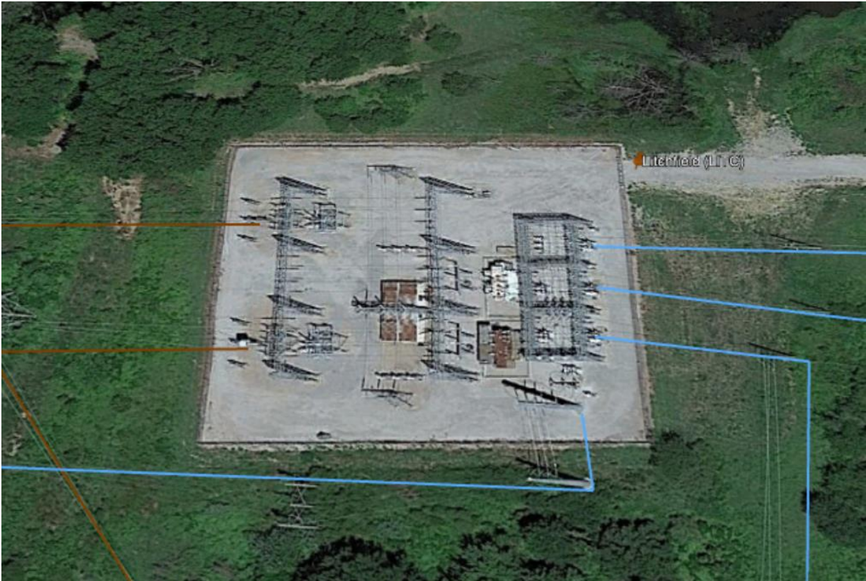
The proposed project for the Network Upgrades is located at Litchfield Substation.
